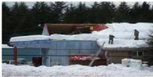
Credit: Ryan McFarland 2009. Collapsed roof
